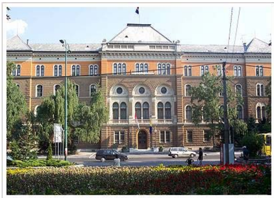
Sarajevo, Governmental Building (1886)
