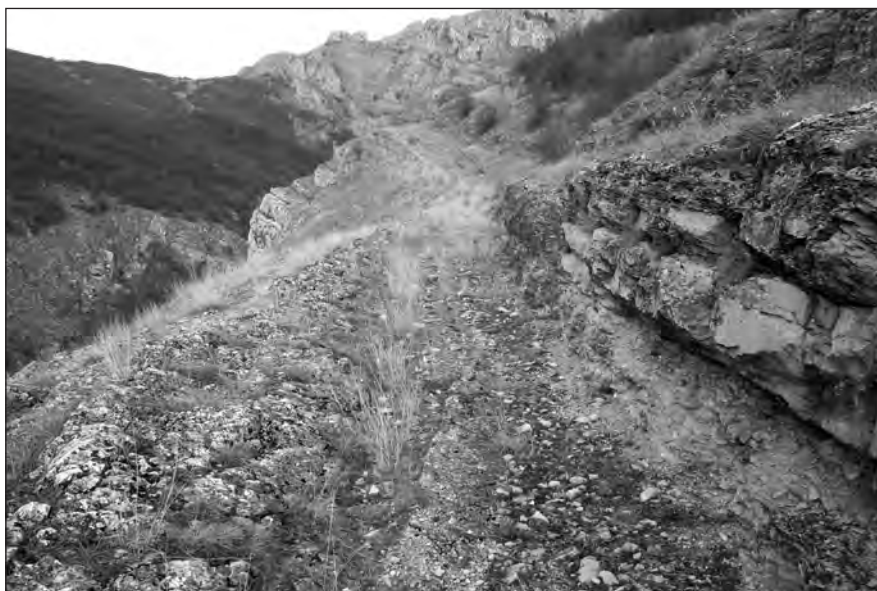
Fig. 1 Remains of the road with visible embankments at the entrance to the Svrlijski Timok gorge
